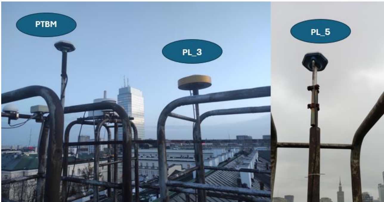
Figure 3-5 PTBM antenna installation at GUM
