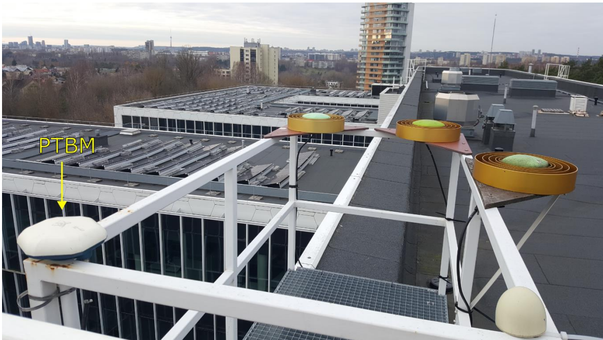
Figure 3-5 PTBM antenna installation at FTMC
