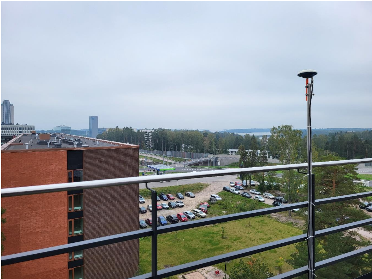
Figure 3-5 PTBM antenna installation at VTT
