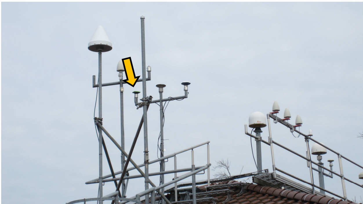
Figure 4-3: Installation of GNSS antennas at PTB, UA04 antenna (orange arrow)
