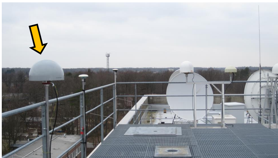
Figure 4-3: Installation of GNSS antennas at PTB Meitner-building, JV03 antenna (orange arrow)
