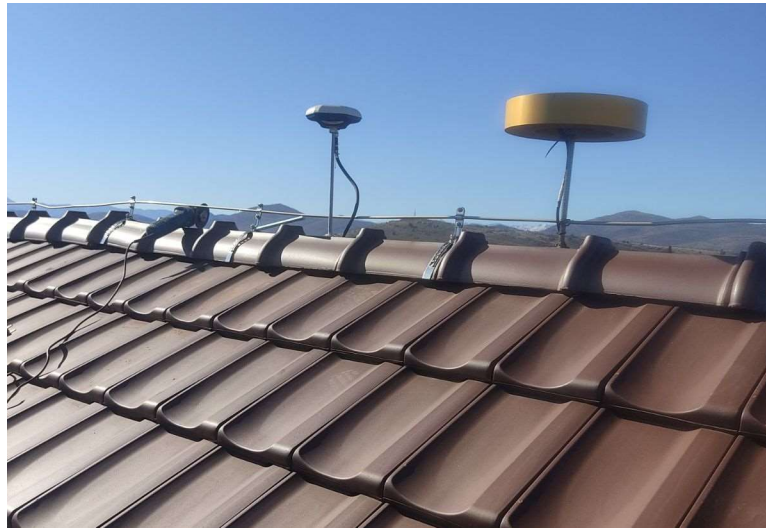
Figure 6-2 Antenna installation on the roof of the MBM building (PTBM left)
