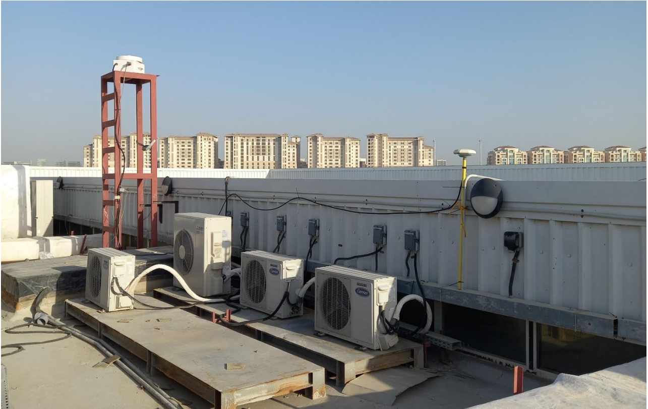
Figure 6-2 Antenna installation at EMI
