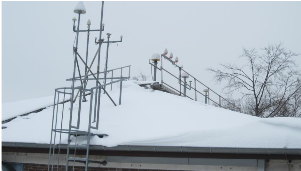
Figure 7-3 Roof conditions at PTB at nominal start of campaign CC2
