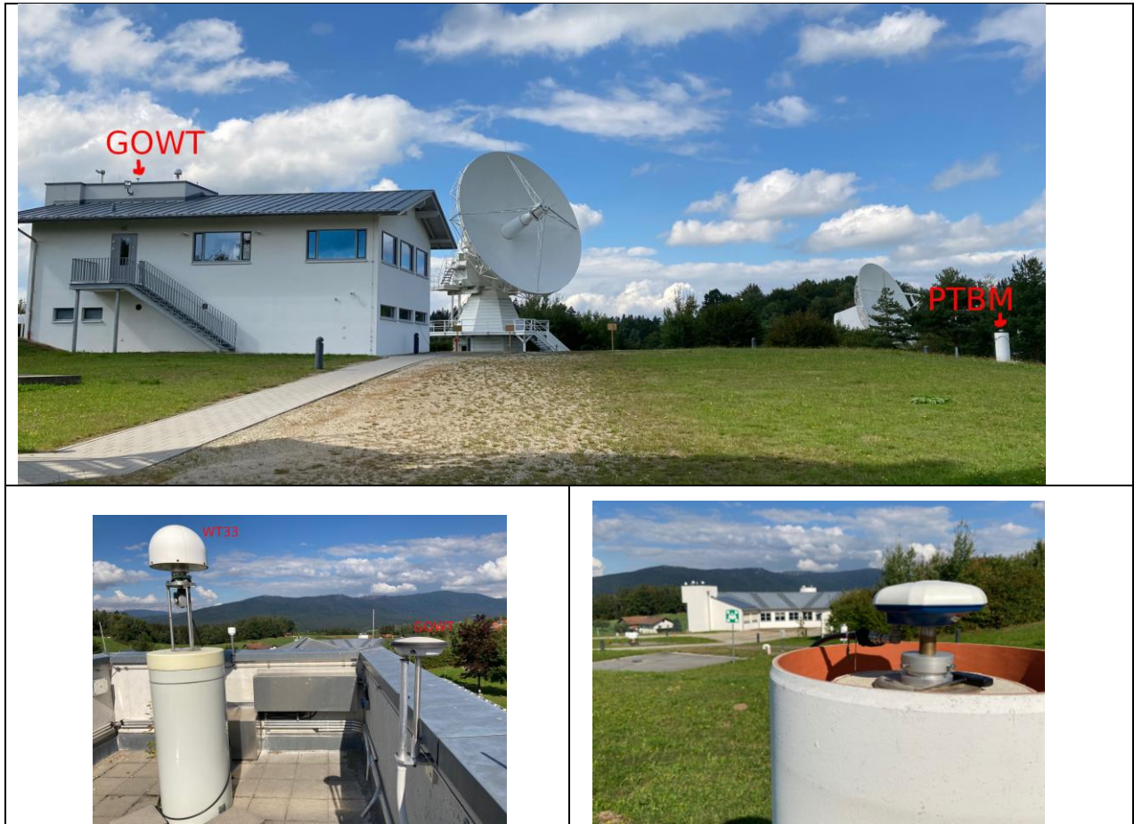
Figure 6-4 GNSS antennas GOWT and PTBM on the GOW area
