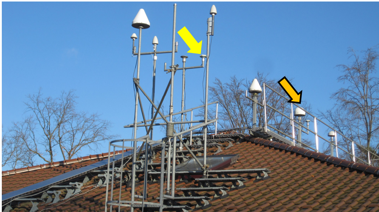
Figure 4-3: Installation of GNSS antennas at PTB
