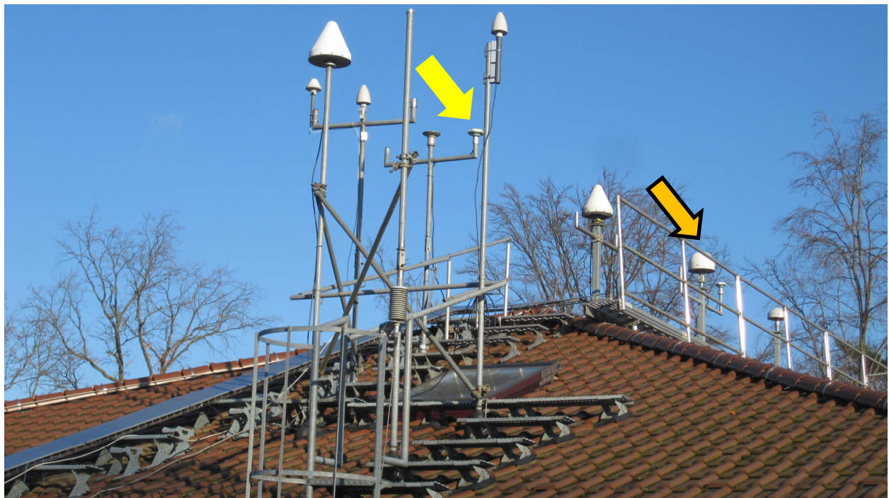
Figure 4-4: Installation of GNSS antennas at PTB
