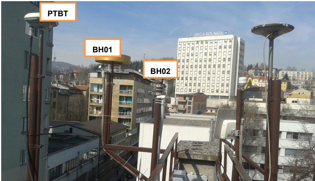
Figure 6-2: Antennas position on the rooftop of the IMBH building
