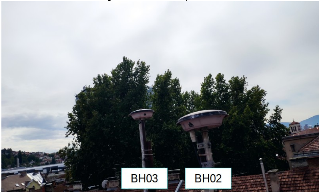
Figure 2: Antenna roof positions
