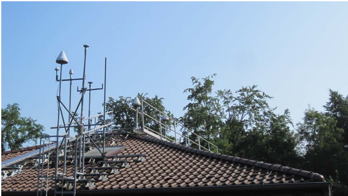
Figure 4-4: Installation of GNSS antennas at PTB
