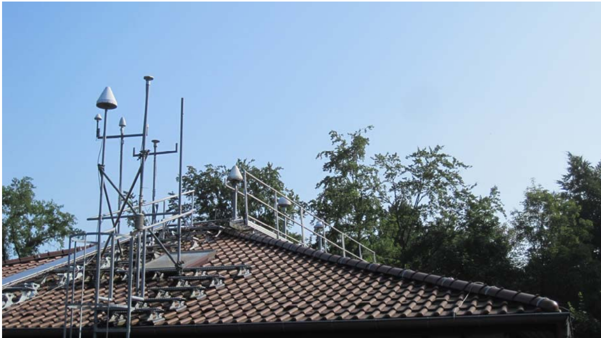
Figure 4-4: Installation of GNSS antennas at PTB
