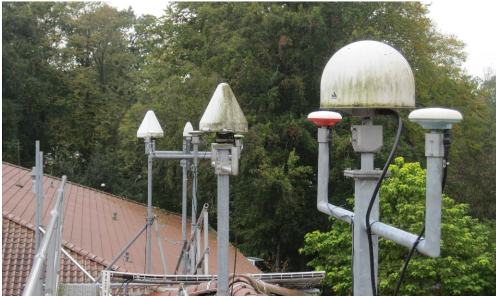
Figure 4-4: Installation of GNSS antennas at PTB
