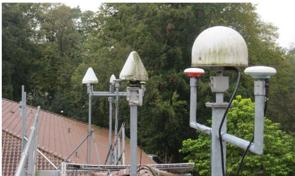
Figure 4-4: Installation of GNSS antennas at PTB
