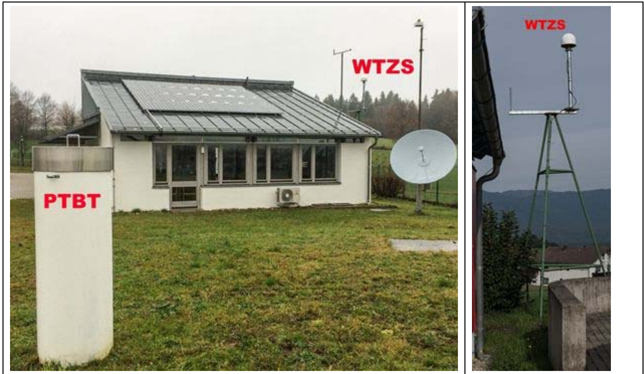
Figure 6-2: Antenna position on the GOW campus and on the rooftop of the GOW building
