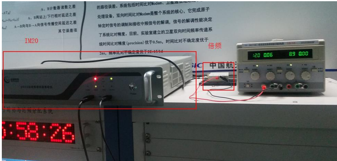
Figure 3. Calibrator installed in BIRM
