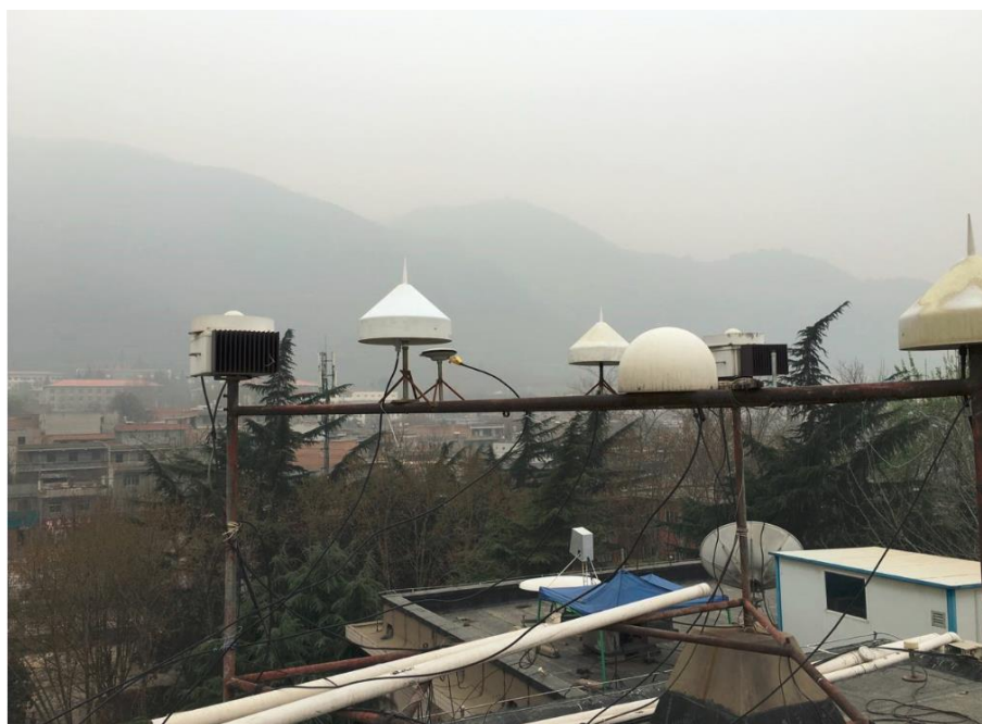
Figure 3. Calibrator installed in NTSC
