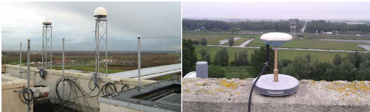
Figure 8-2: Installation of GNSS antennas on the VSL roof: from left to right: VSLG, VSLF, and PTBT
