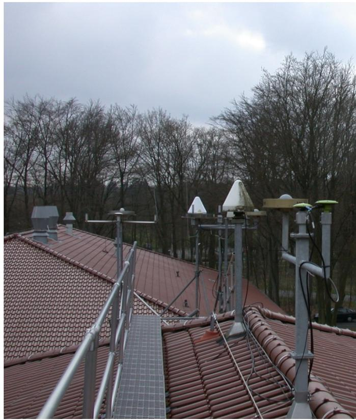
**Figure 4-4: Installation of GNSS antennas at PTB**
