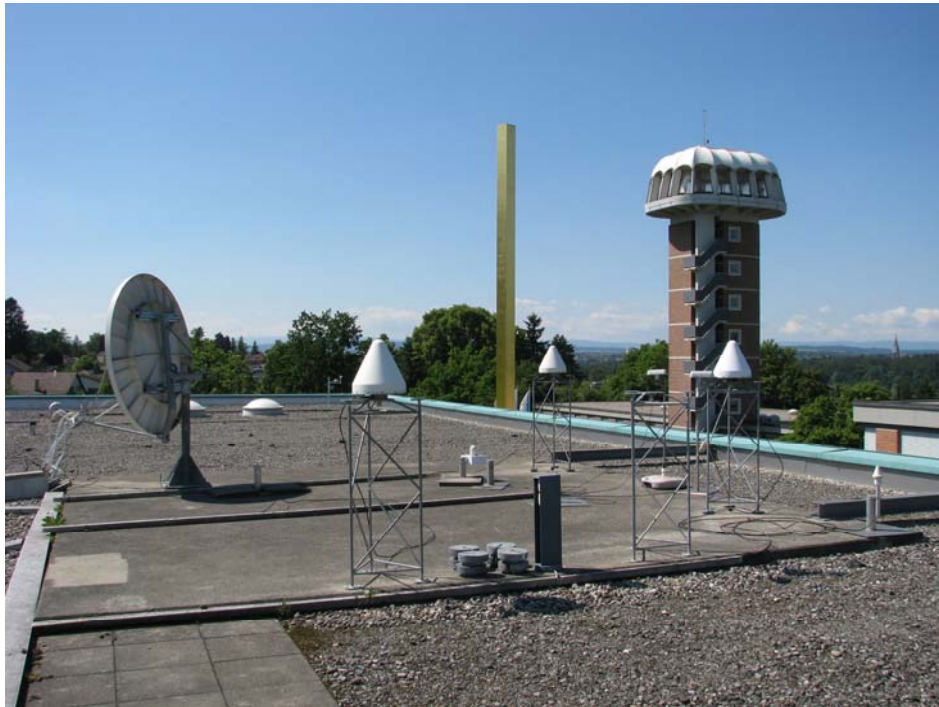
Figure 7-2: Installation of GNSS antennas on the METAS roof
