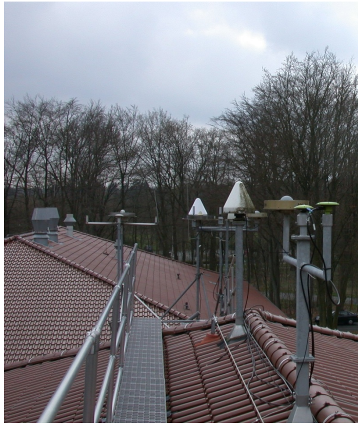
Figure 4-4: Installation of GNSS antennas at PTB
