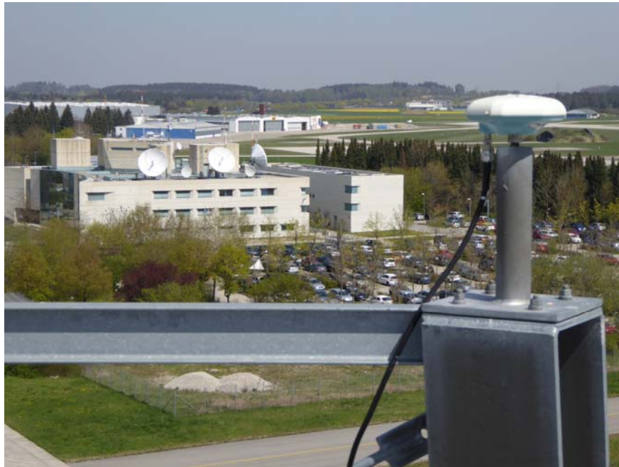
Figure 6-2: Installation of the PTBT antenna on the DLR IKN antenna rack
