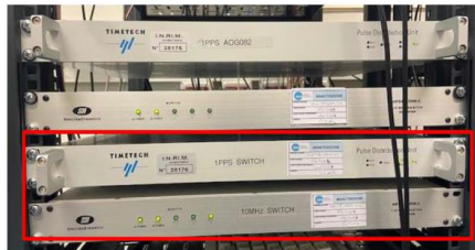
UTC(IT) TF signals Distribution at Time Lab. towards the RadioNavigation Lab. (TimeTech Pulse Distribution Unit and SDI HPDA-15RM-C)
